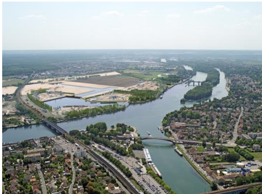
The PSMO on completion of development phase 1 (2024/2027) – aerial view
